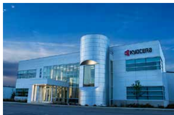
KSPT Round Tool Mfg. Facility Ohio (USA)
