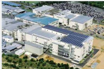
KYOCERA Corp. Indexable Mfg. Facility Yokaichi Facility (JAPAN)
