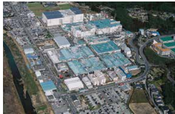
KYOCERA Corp. Indexable Mfg. Facility Sendai Facility (JAPAN)
